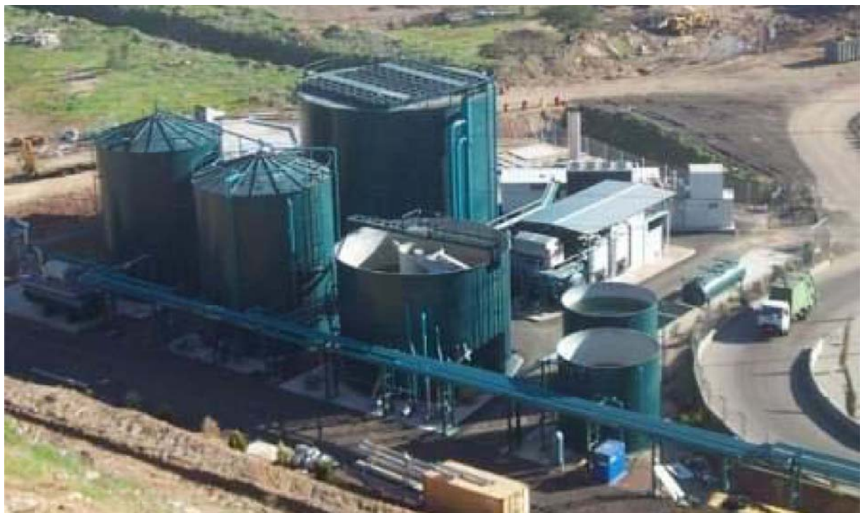
A large sized Bio Gas Plant to produce about 36,000 Cub M per day
